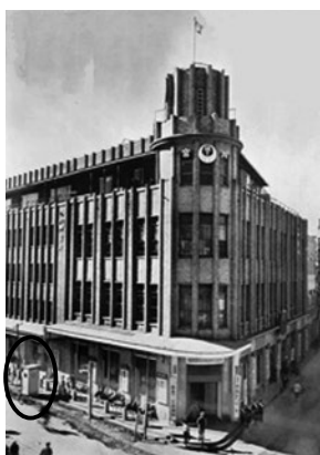
[fig.6] Miyagawa Departmentstore. source: http://www.mutusinpou.co.jp/ まちネタ散歩! 陸奥新報(続々)
